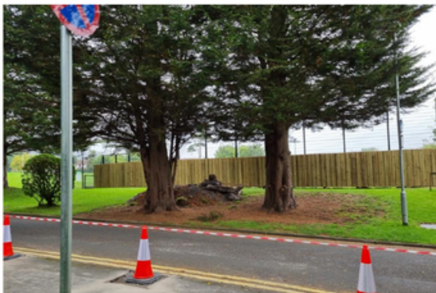
Fencing from footpath north of school access
