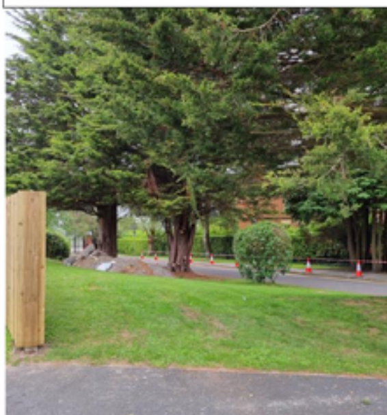
View within the site from acoustic barrier towards the boundary with Nos. 2 & 4 Belfast Road
