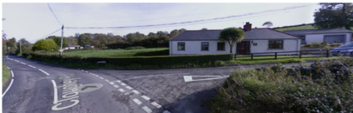
Figure 1: Google image of the two 'frontages' along Ballygalget Road and Cloughey Road
