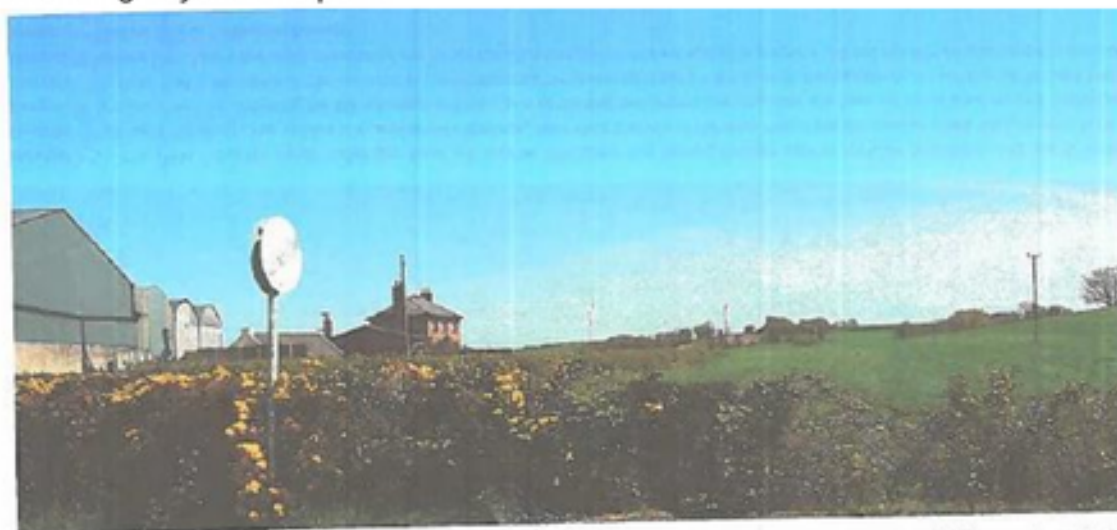
From this vantage point, the crossroads at Kilmoor Church and Lisbarnet Roads, the proposed turbine is not highly conspicuous in the
