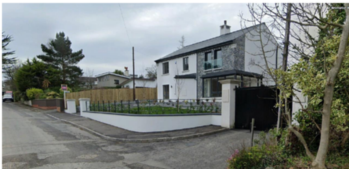
View of House 1 to front of site looking back up Brompton Road
