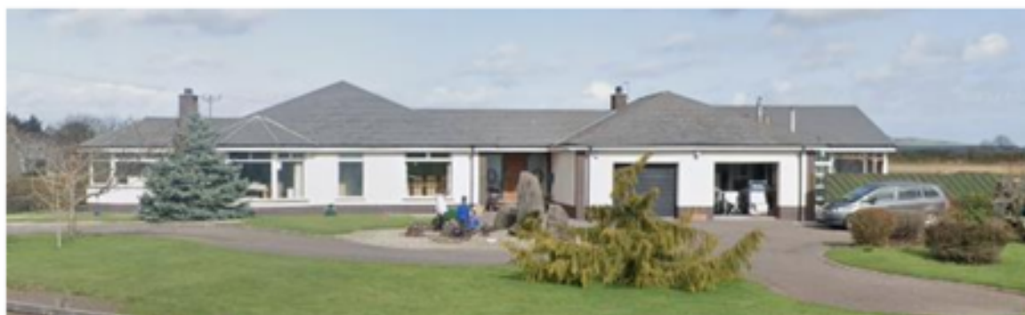
No. 83 with attached double garage
