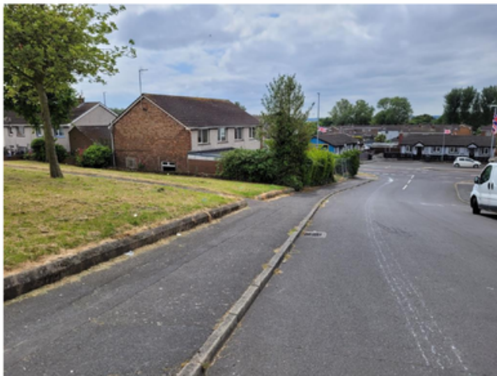
Photograph of site on the corner. Taken on Queen Street looking towards Upper Greenwell Street
