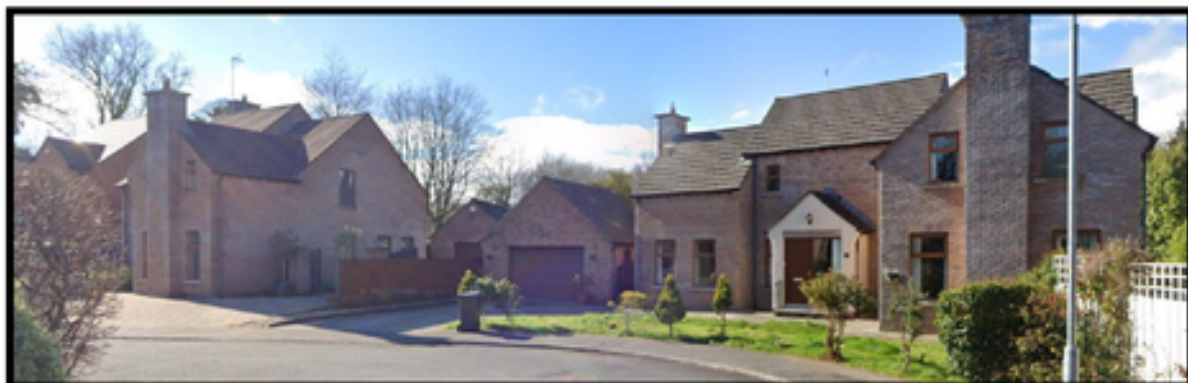
Front elevation of dwelling.
