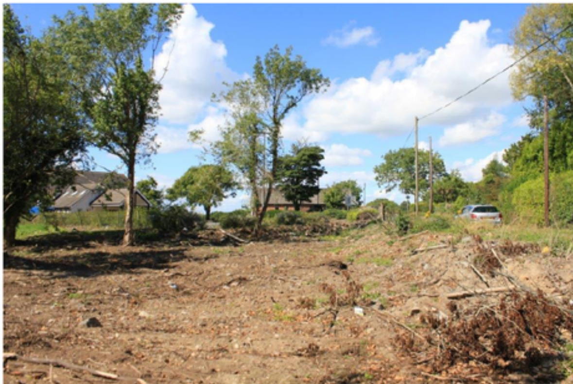
Figure 9 – View of site from east
