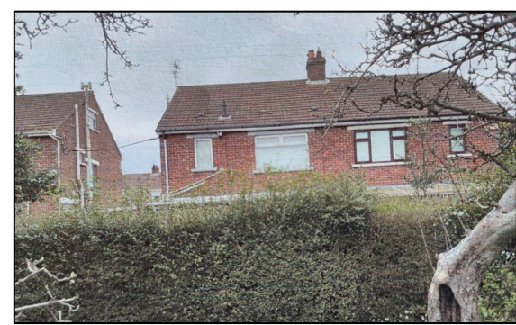
Figure 5 – Existing dwellings to the rear
