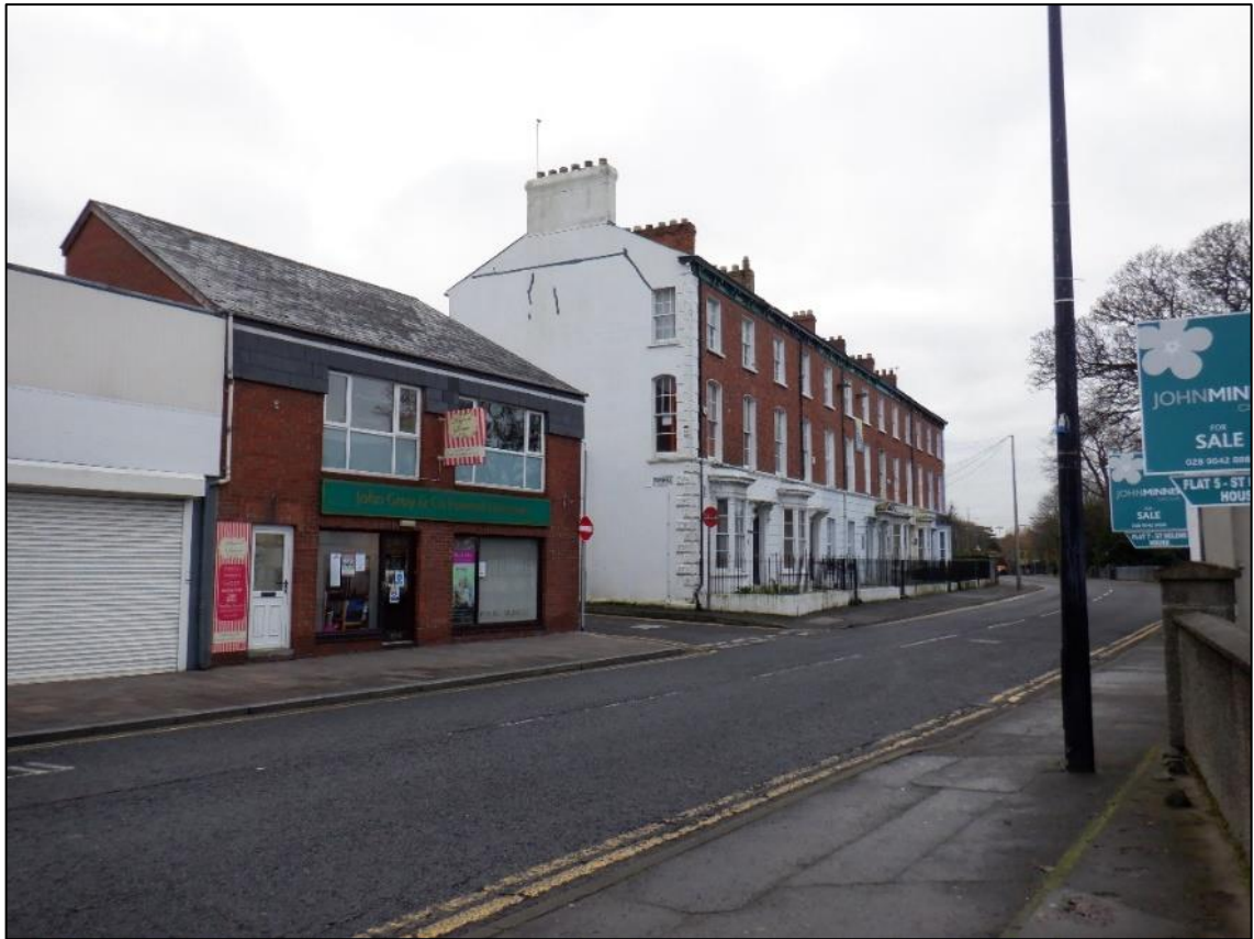
Figure 8 - Existing 3 storey buildings to south of site
