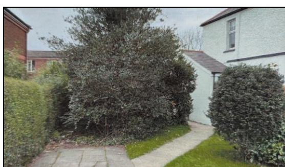
Figure 3 – Side of existing dwelling
