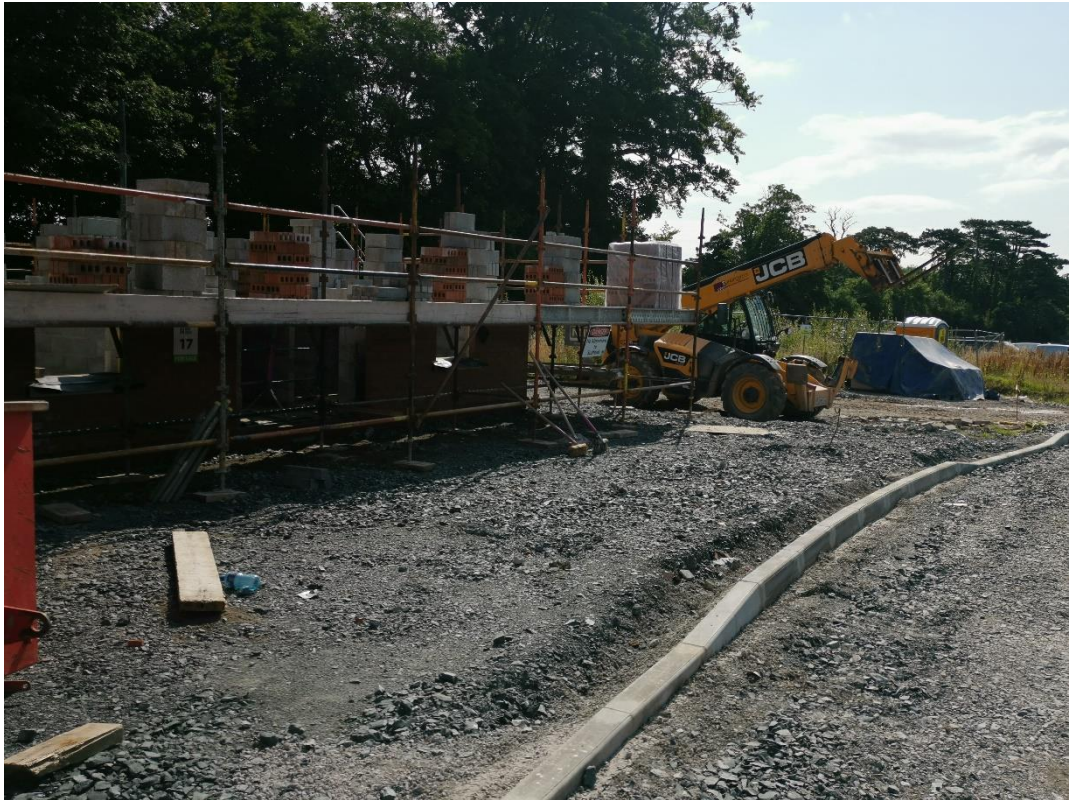
Photo 3: View towards application site with adjacent dwelling no17 under construction (left)
