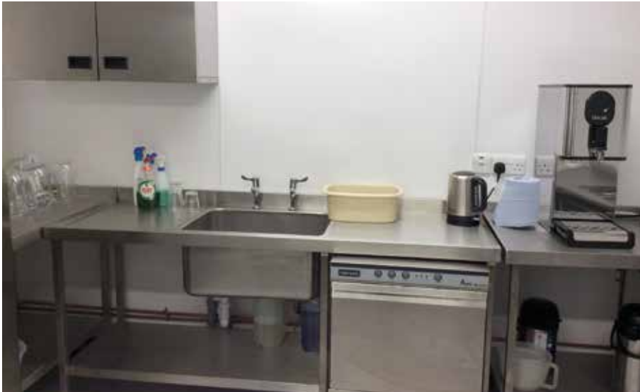
New kitchen facilities installed at Portavogie Community Centre
