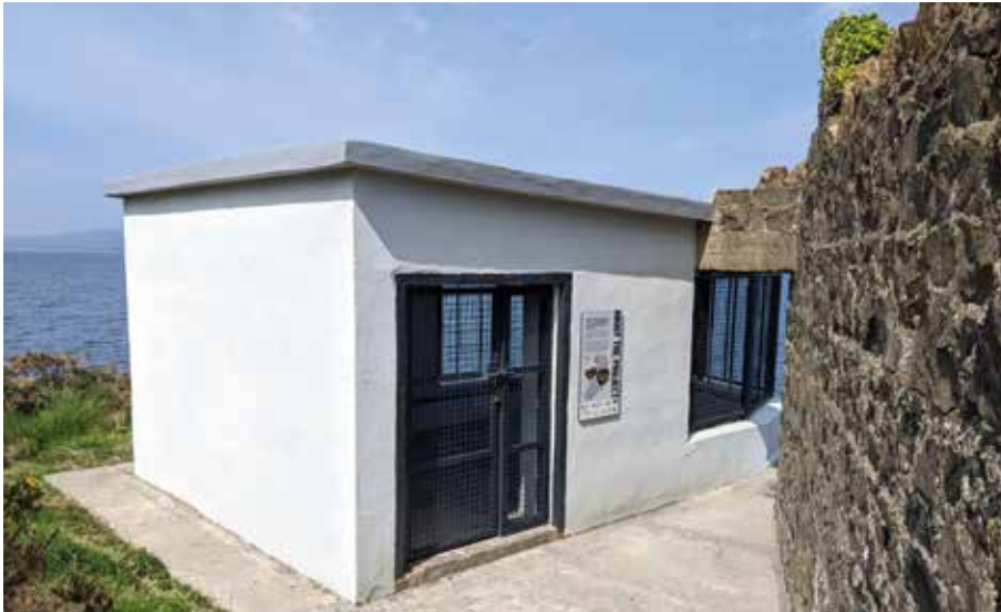
One of the 3 refurbished searchlight emplacements
