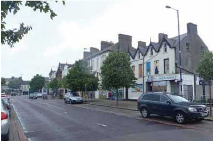
Existing Building Terrace along Queen's Parade
