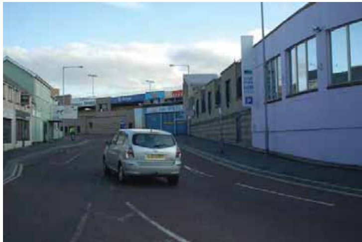
Flagship Centre façade requiring improvement
