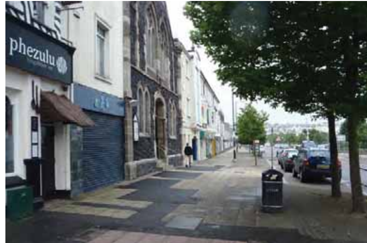
Existing Public Realm - Variation in Street Pavements / Footpaths
