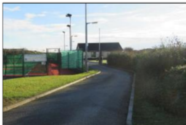
Figure 1 – View of site from access road
