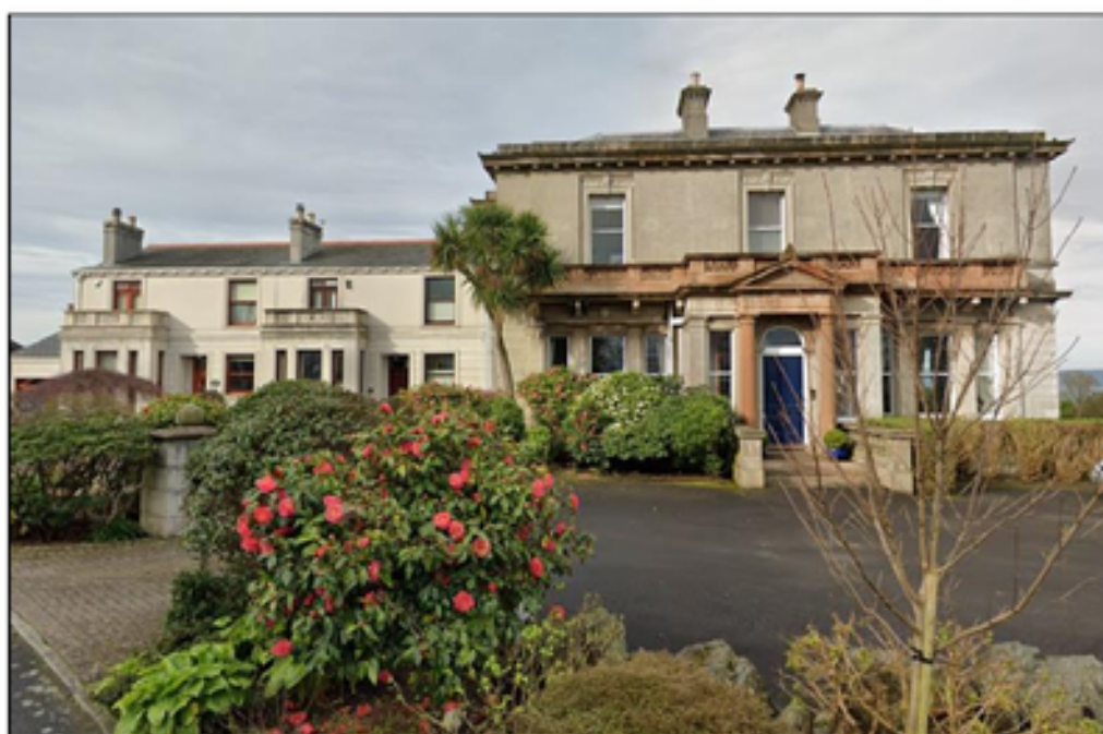
Figure 29 - View of Nos 1-4 Seacourt
