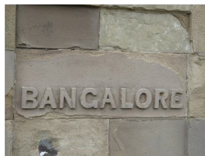
Fig.12 - Delamination
