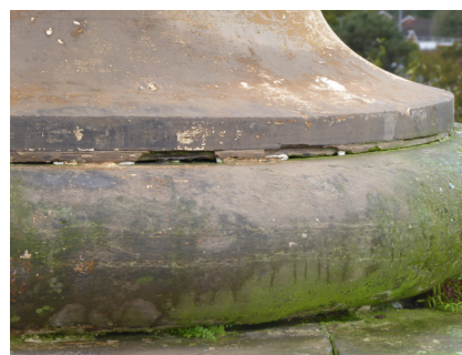
Fig.27 - Fracture
