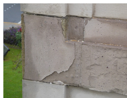
Fig.21 - Delamination
