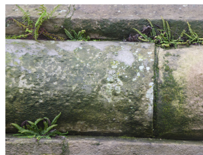
Fig.20 - Algae and lichen soiling
