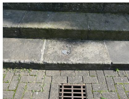
Fig.39 - Patch repair
