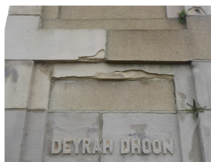
Fig.35 - Delamination
