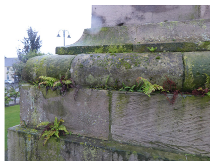
Fig.32 - Vegetation growth in open joints
