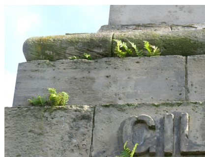
Fig.41 - Algae and vegetation in open joints
