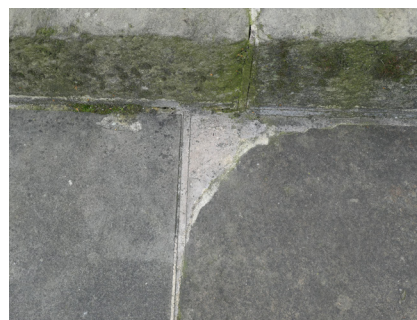
Fig.29 - Putty lime pointing
