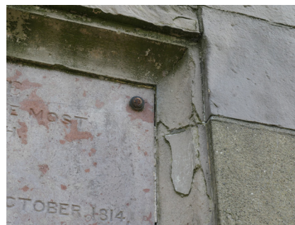
Fig.40 - Delamination
