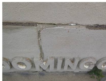
Fig.34 - Delamination
