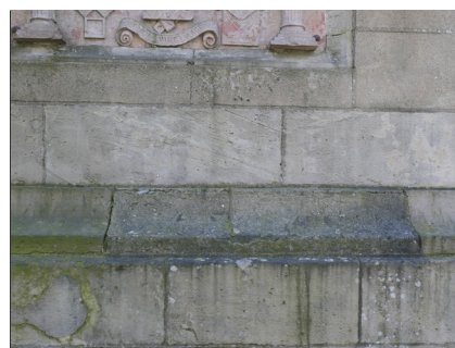
Fig.07 - Cementitious mortar repairs
