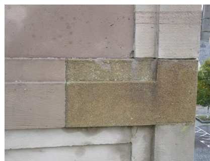
Fig.42 - Cementitious mortar repair
