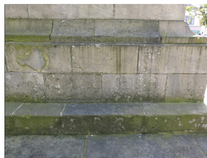
Fig.06 - Algae and lichen soiling
