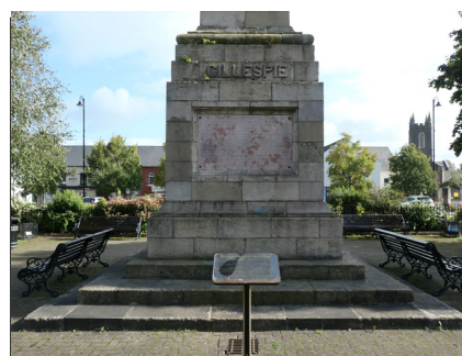
Fig. 1 - Stepped base and pedestal
