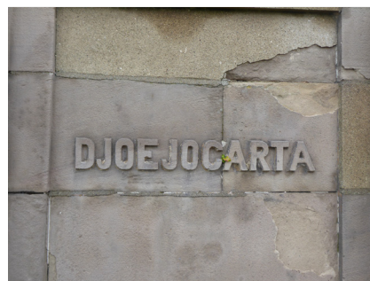
Fig.44 - Delamination
