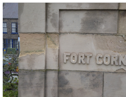
Fig.24 - Extensive delamination
