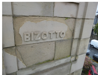
Fig.23 - Extensive delamination
