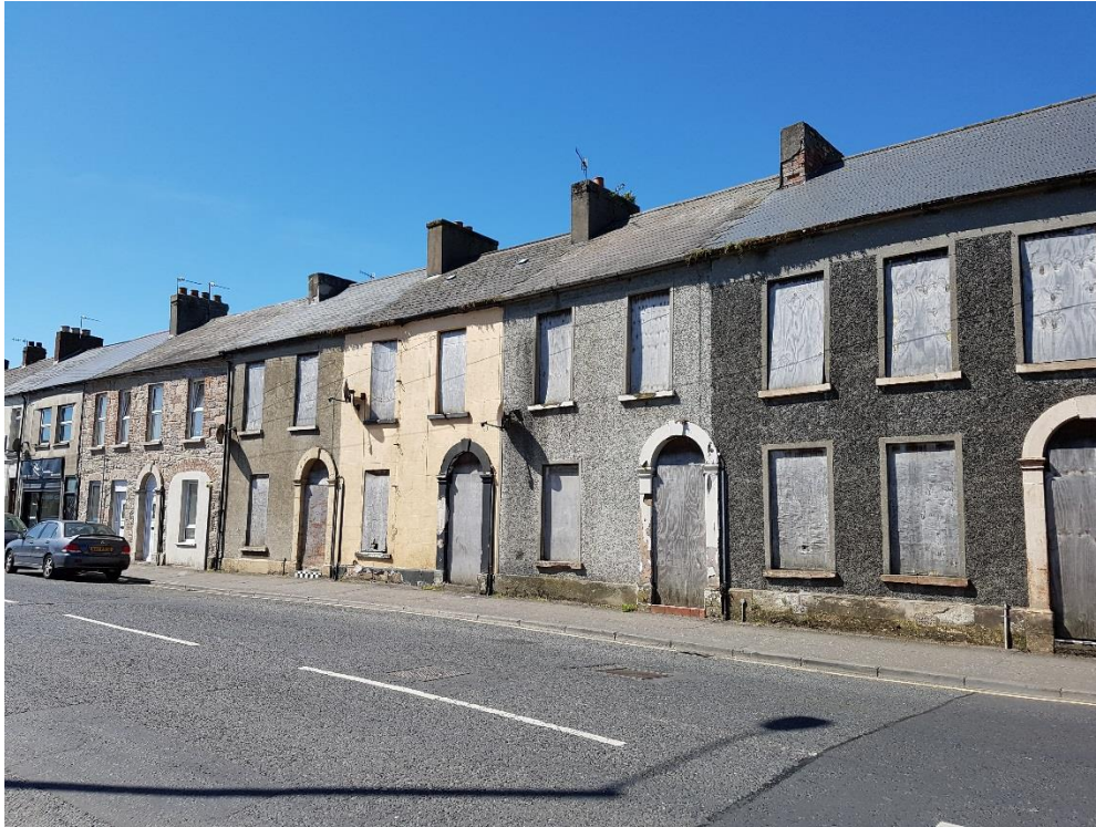
Figure 7: Dereliction in South Street
