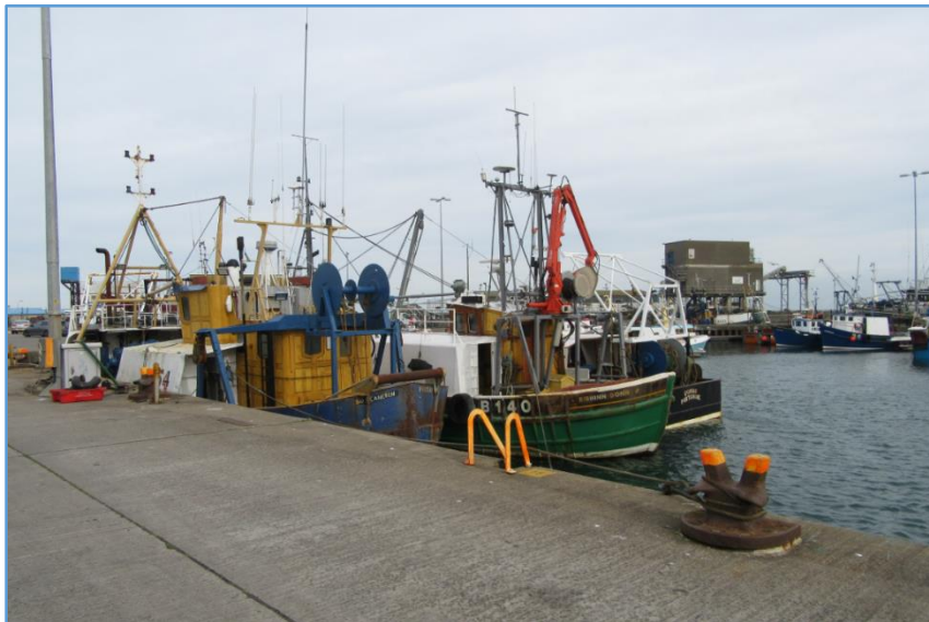
Photo 5: Portavogie Harbour. Source: Ards and North Down Borough Council
