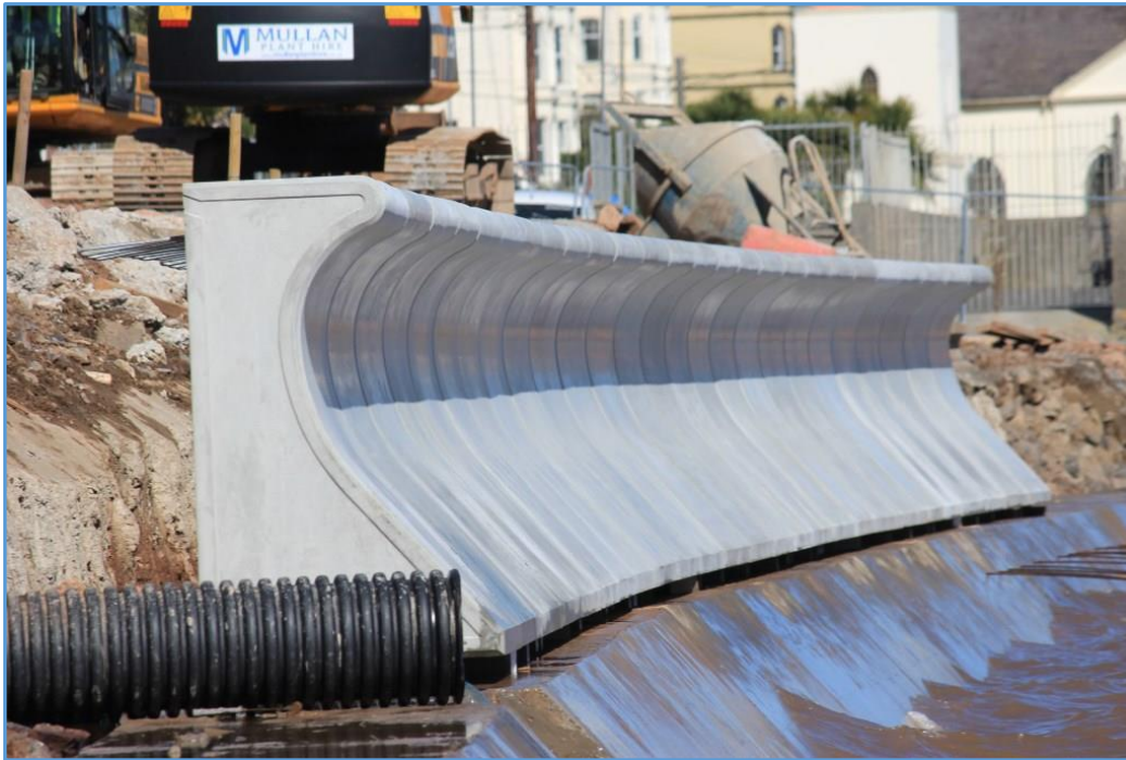
Photo 8: New coastal defences were put in place in Donaghadee as part of the public realm works in 2015.
