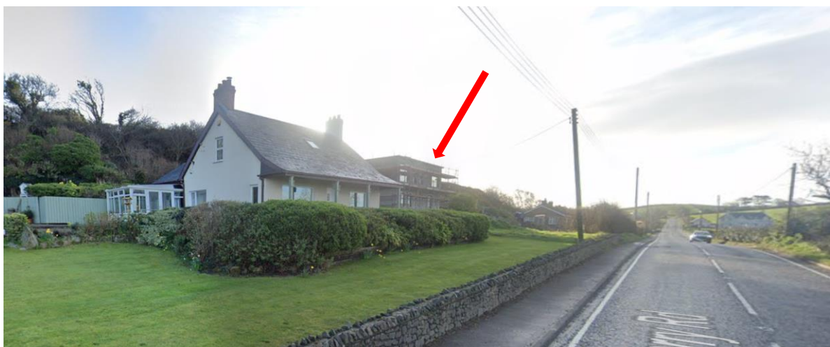
Google Street view Image March 2023 showing approved dwelling under construction.
