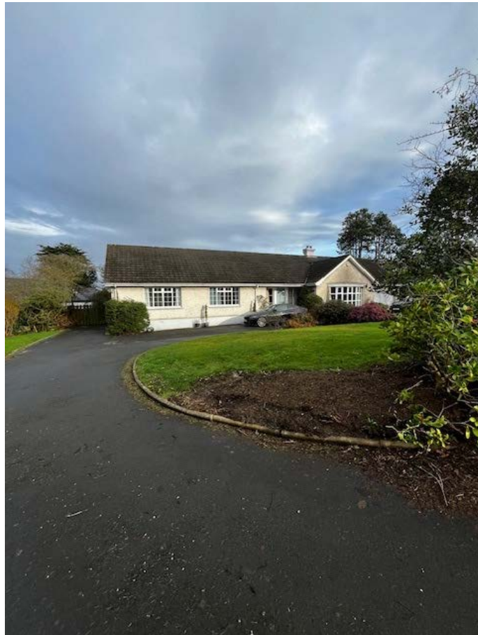
Front of existing dwelling
