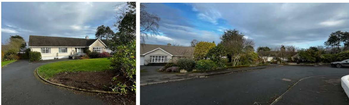
Figure 4: Existing dwelling to be replaced
