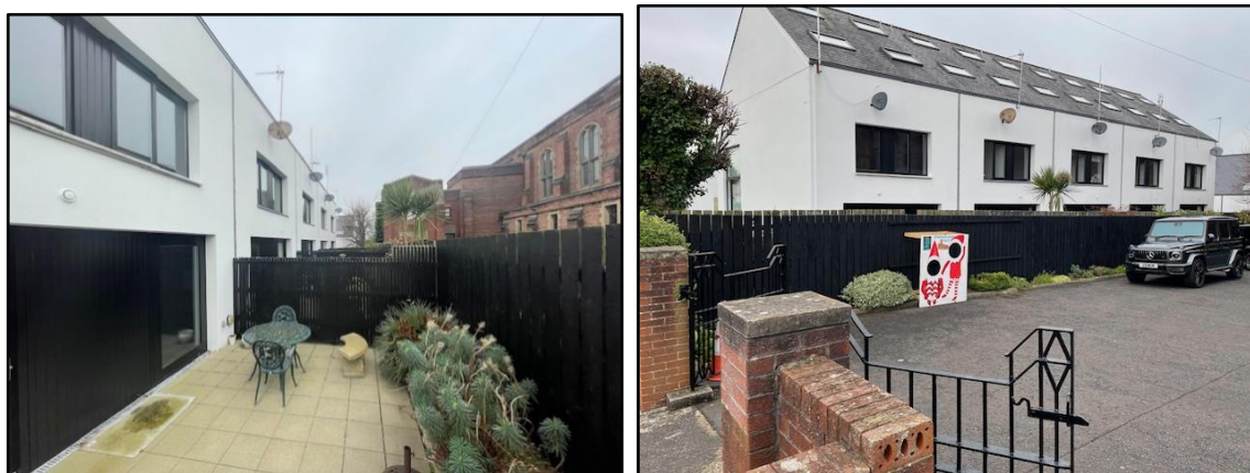
Figure 4 - Photos of rear elevation of terrace
