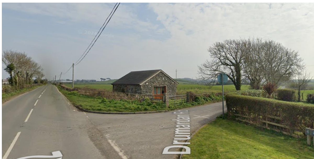
Existing building to be converted.
