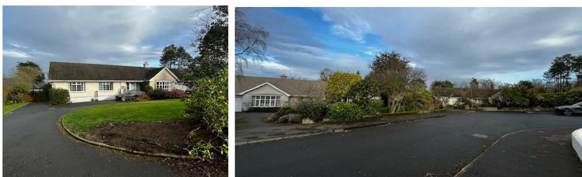
Figure 4: Existing dwelling to be replaced
