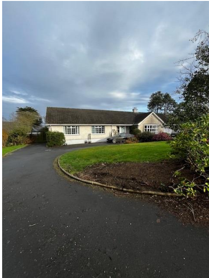
Front of existing dwelling
