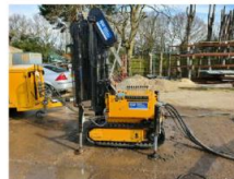
Mini-Pile machine for drilling to avoid damaging neighbouring structures
