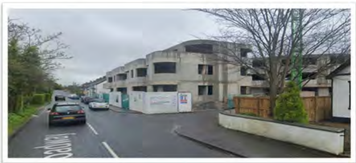
Apartments now nearing completion on Broadway
