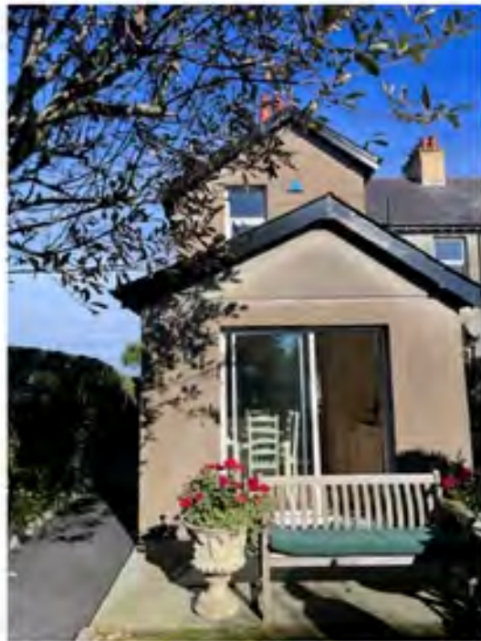
Patio doors to rear of No. 17
