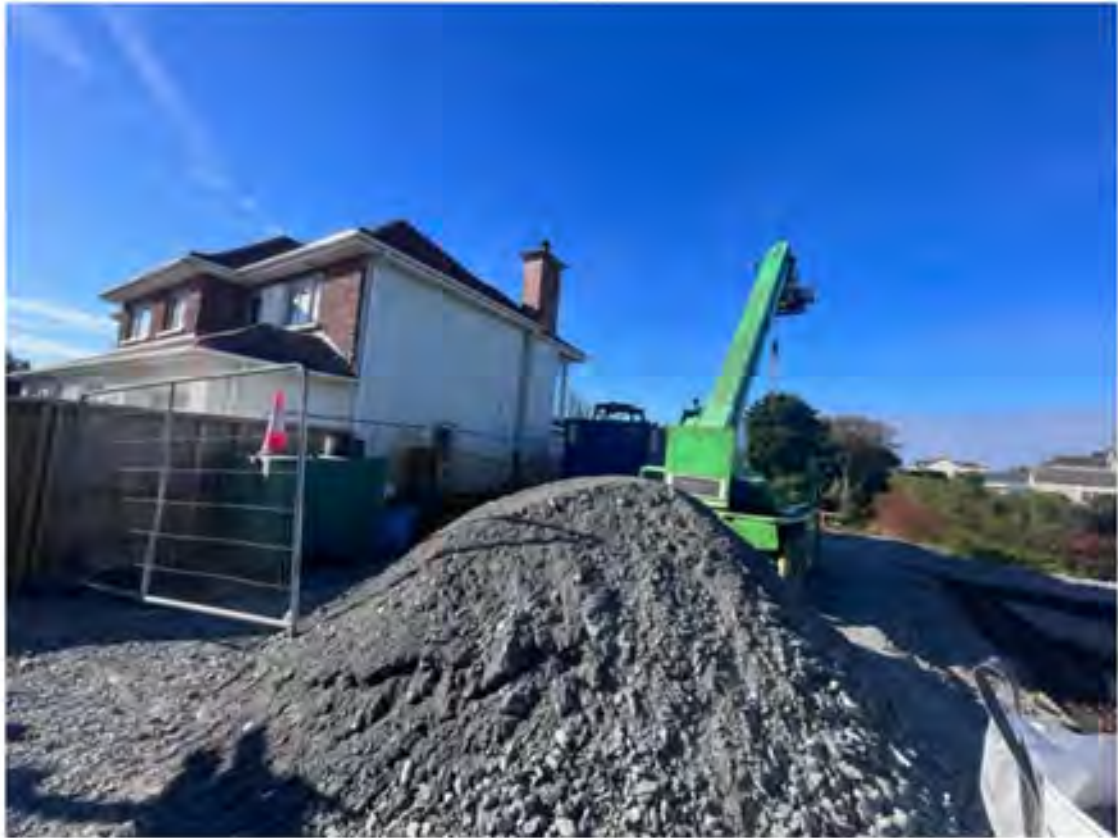
No. 15 Morningside to rear of site
