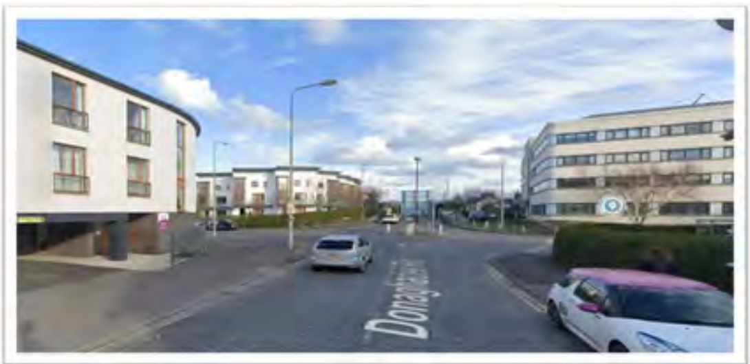
Multiple Apartment Blocks at junction of Donaghadee Road and Hamilton Road
