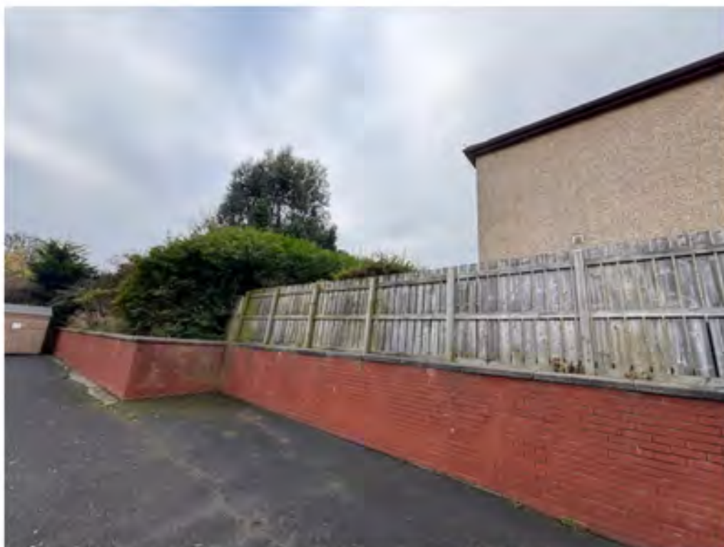
View towards site from side of Towerview Gardens
