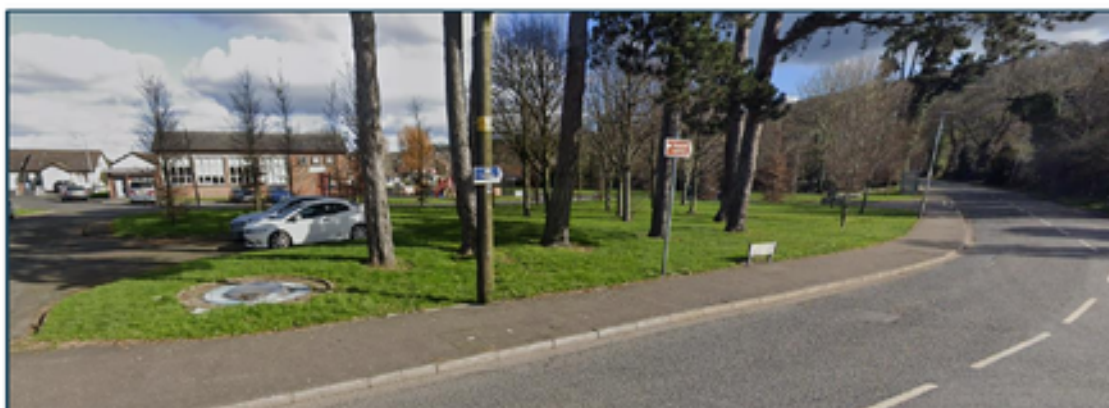
View from main road through trees towards the subject building
