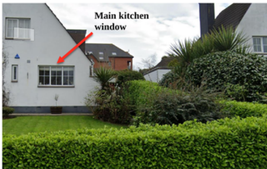
Figure 10 – Main front facing kitchen window to 17A
