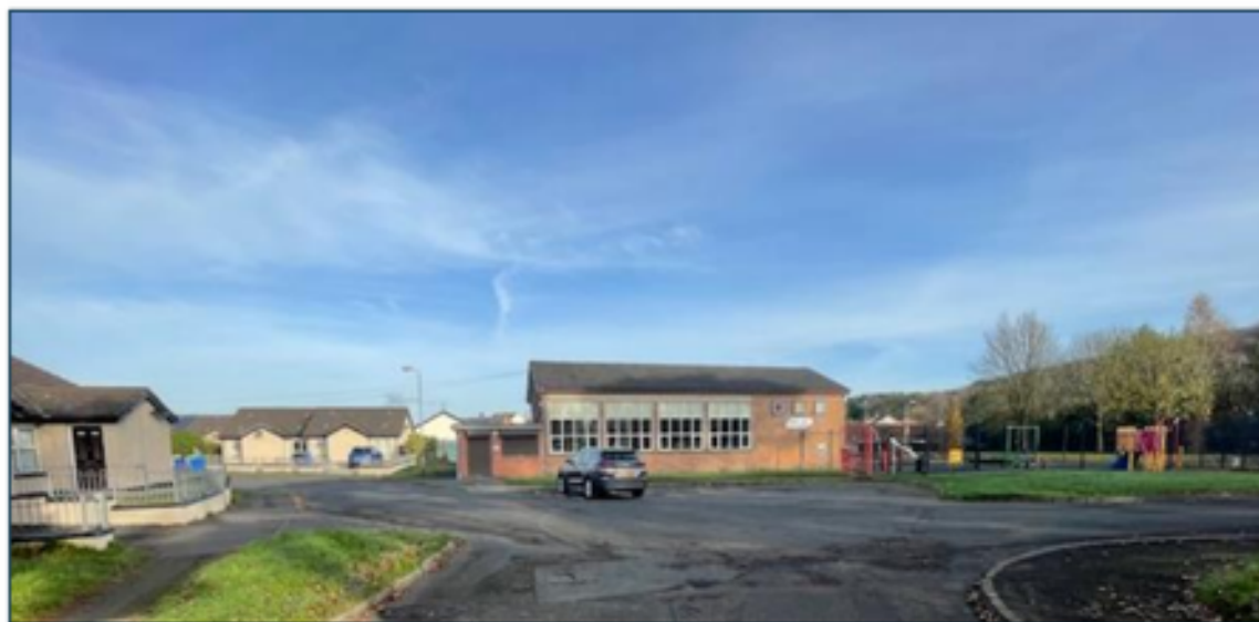
Main view of the front of the building
