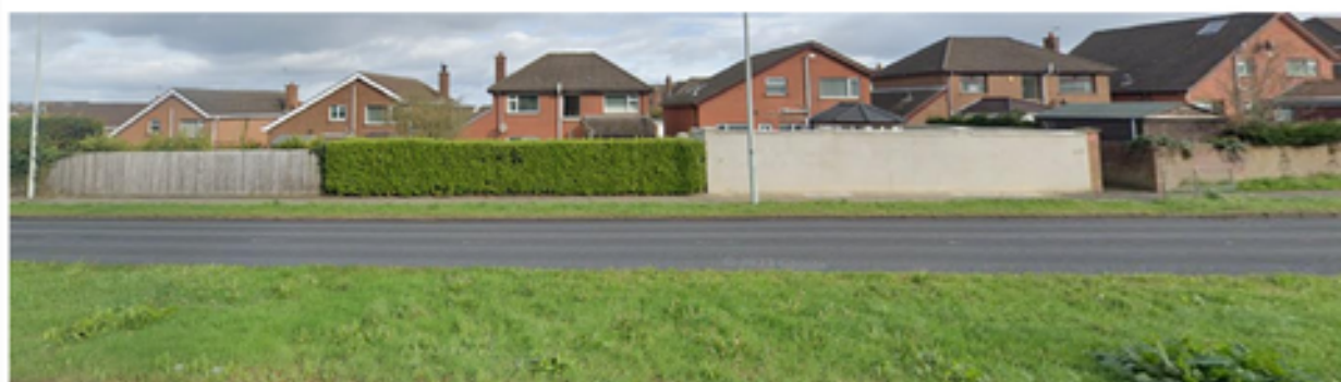
Fig 8: Image from Google Street View showing dwellings in Cleland Park South when viewed from the carriageway (March 2023)
