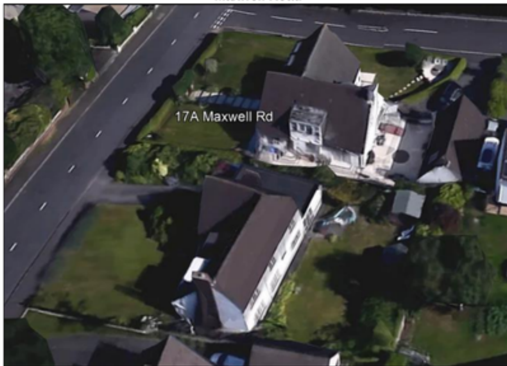
Figure 13: Orientation of Application Dwelling Towards the Double Glazed Doors of No. 17A Maxwell Road
