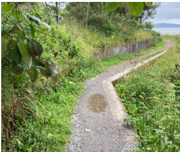
Further along across the frontage of the WWTW
