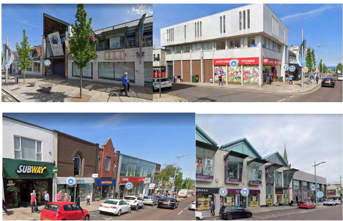
Figure 60 – Examples of modern architecture on Main Street
