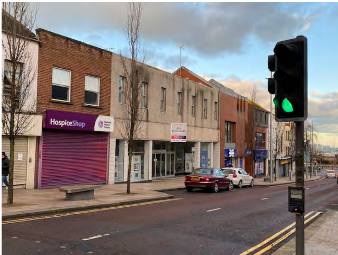
Main Street site frontage
