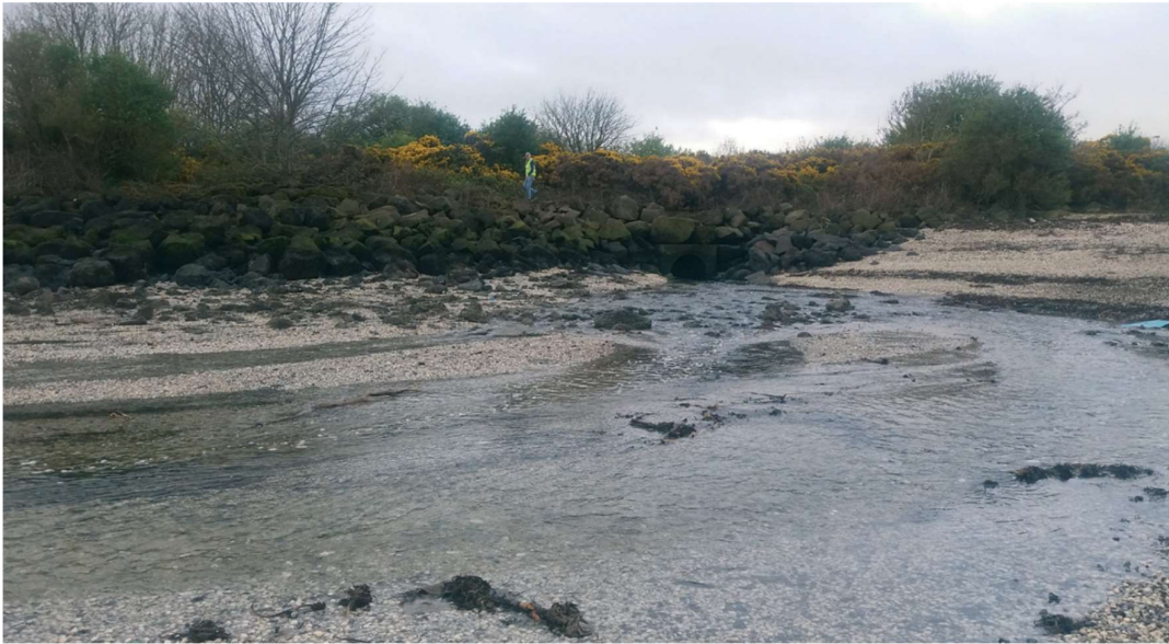
Figure 15: Whitehouse WwTW Discharge Headwall (temporary in 1977)
