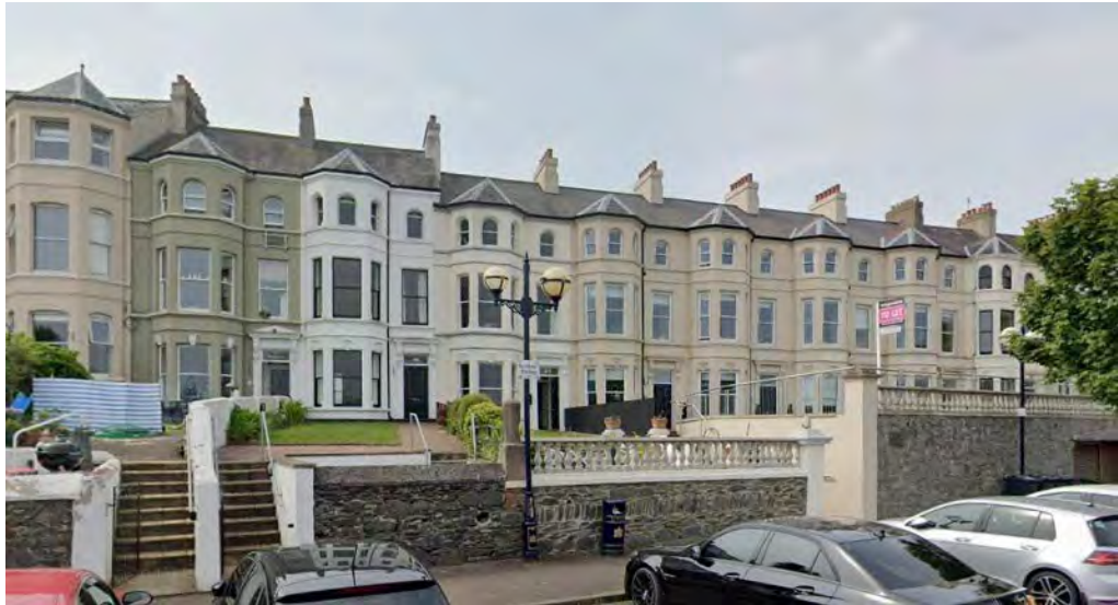
Figure 24 – Existing residential terraces on Queen’s Parade
