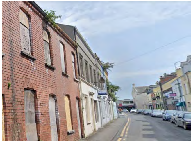
Figure 49 – Terraced Dwellings on King Street
