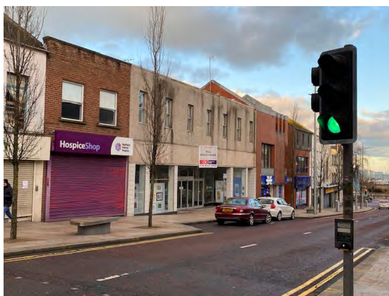
Figure 48 – Existing buildings to be demolished on Main Street
