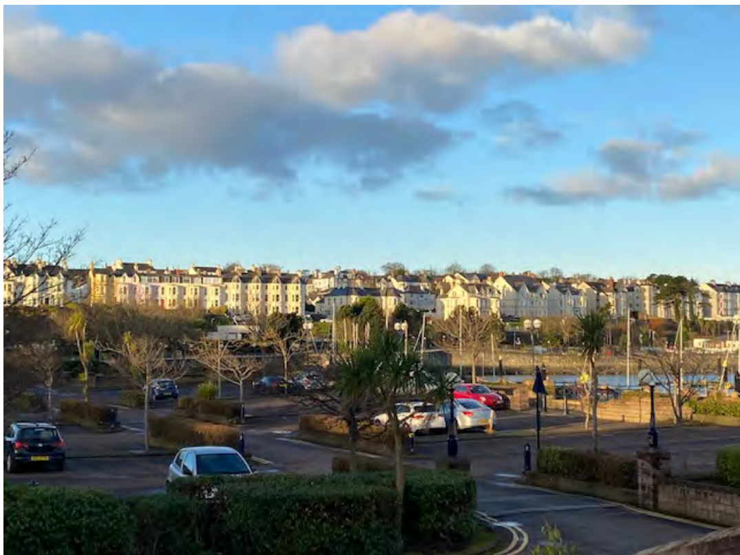
Victorian terraces viewed from Marine Gardens Car Park
