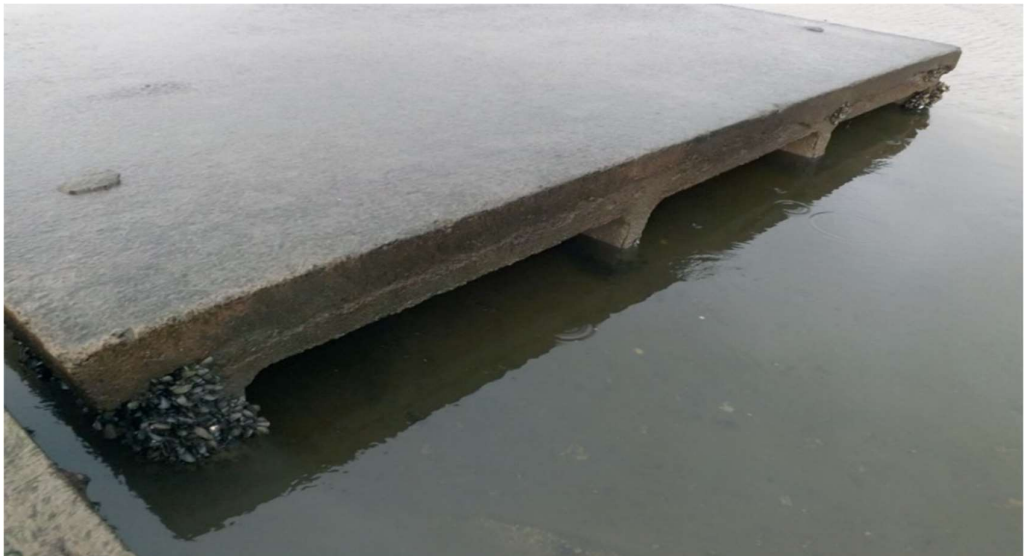
Figure 12: Seaward end of the 7m wide Belfast WwTW Sea Outfall Culvert
