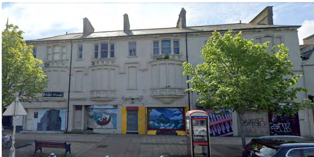
Figure 57 – Existing Buildings at 5-8 Queen's Parade Proposed for Demolition
