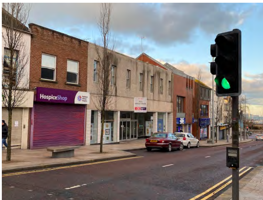
Figure 39 – Existing buildings on Main Street to be demolished
