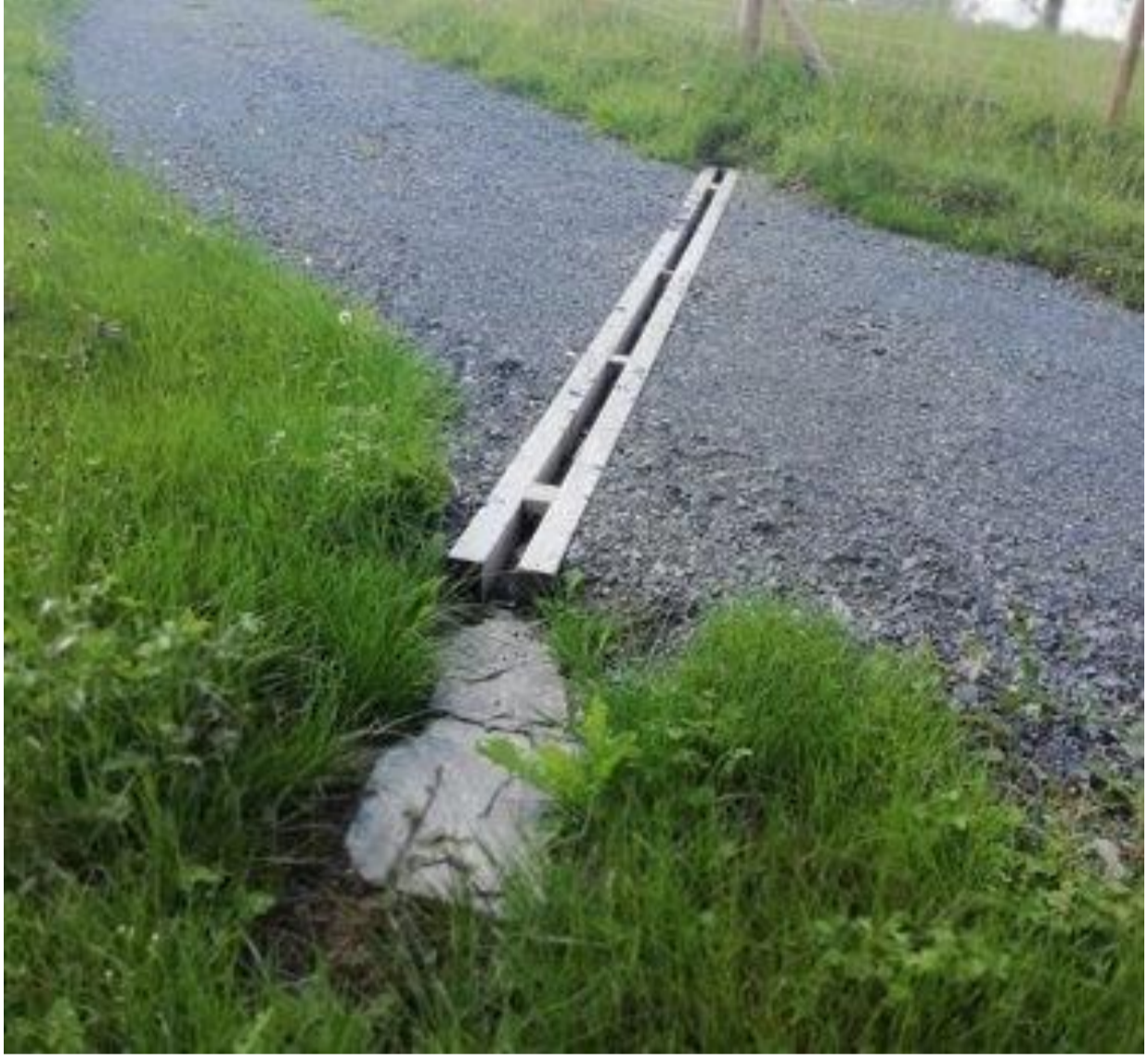
Figure 27: Gravel trail incorporating drainage Waterbar
