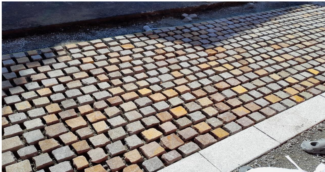
Cobbles being laid outside the Rock Bakery building
