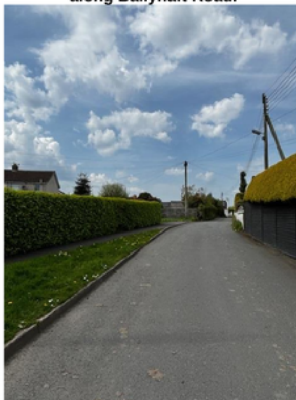
Photo 2: Site is situated in the middle part of this photograph, showing existing boundary wall proposed to be increased in height to 1.8 metres.
