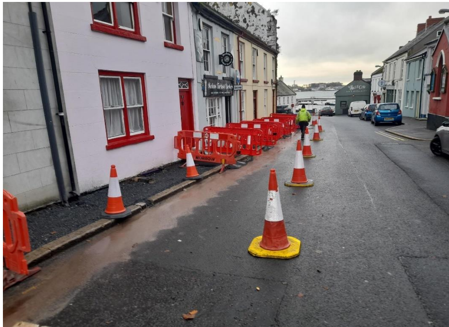
Works begin on Ferry Street
