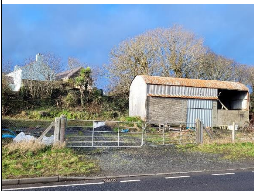
Figure 6 Photograph showing the proposed site and 1 Ballyvester Road to the rear.
