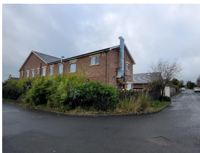
Figure 5 Photograph of the residential home located opposite the site on Bryansburn Gardens.
