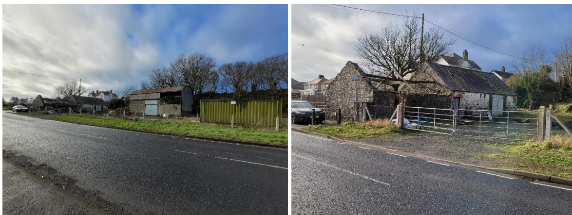
Figure 2 Photographs of the existing stone outbuilding
