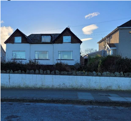
Figure 10 Photograph showing the existing gable elevation to 63 Ballyholme Esplanade.
