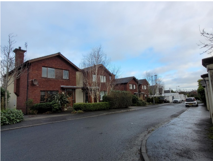
Photograph of the existing semi-detached dwellings in Bryansburn Gardens
