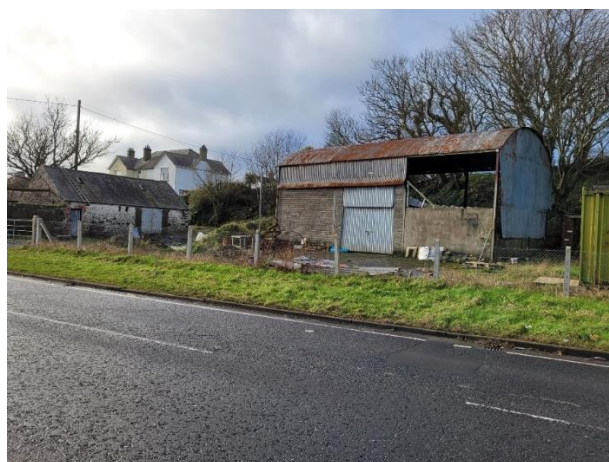
Figure 3 Photographs of the structure to be replaced
