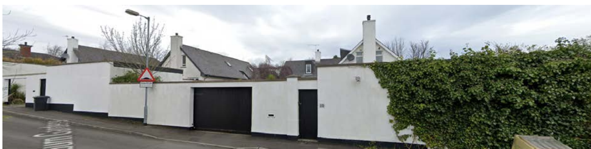
Figure 2 Existing dwellings on Bryansburn Gardens
